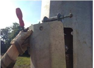
I. After all the necessary job on luminaries is done, start to wind the rope using hand winch and bring the pole to its original (closed) position. If needed, we are helping with the hand rope and keeping this one tensioned all the time. Be careful by this operation, to avoid some own-closing effect, that could cause closing the pole from 2-3m before reaching the end-point and could cause vibrations and some accident.
